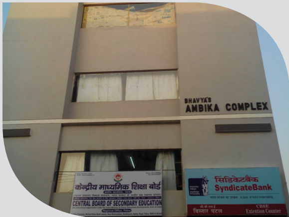
Regional Office & COE Patna Anibika Complex, Behind State Bank Colony Near Brahmsthan Sheikhpura, Raza Bazar, Bailey Road, Patna, Bihar-800014
