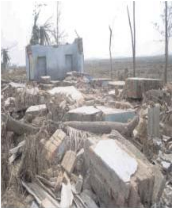
A school building lies in shambles after the cyclone, wind and water ravaged the village
